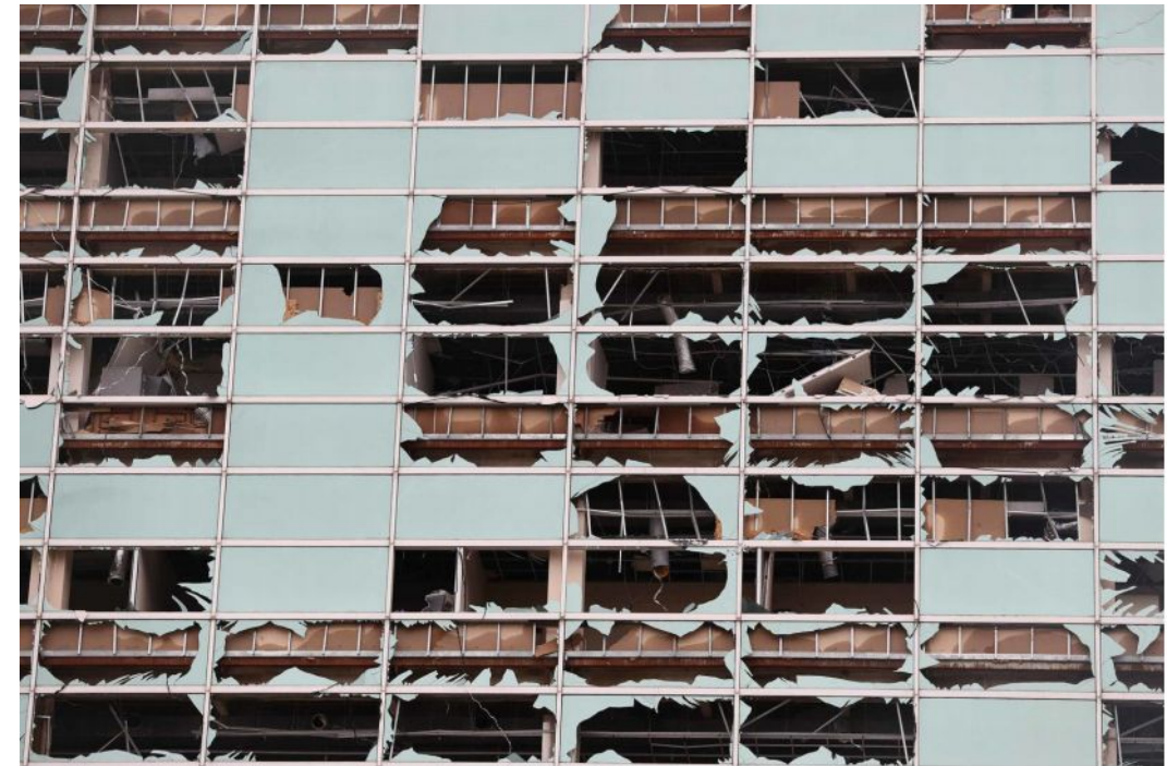
Figure 14. Windows blown out of the Capital One Tower in downtown Lake Charles after Hurricane Laura. Joe Raedle/Getty Images.
